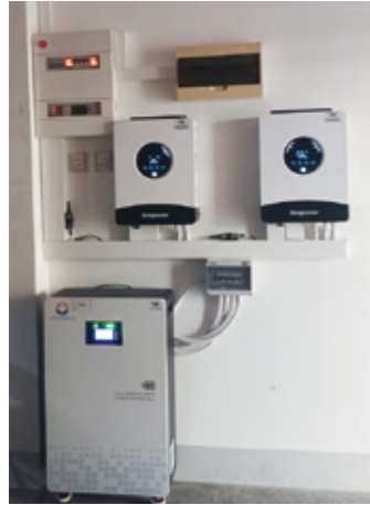
12KW System in Yangon Myanmar 🇲🇲
