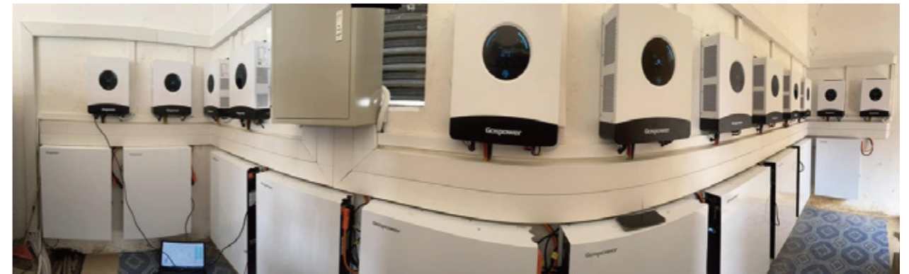
72KW System in Yangon, Myanmar 🇲🇲
